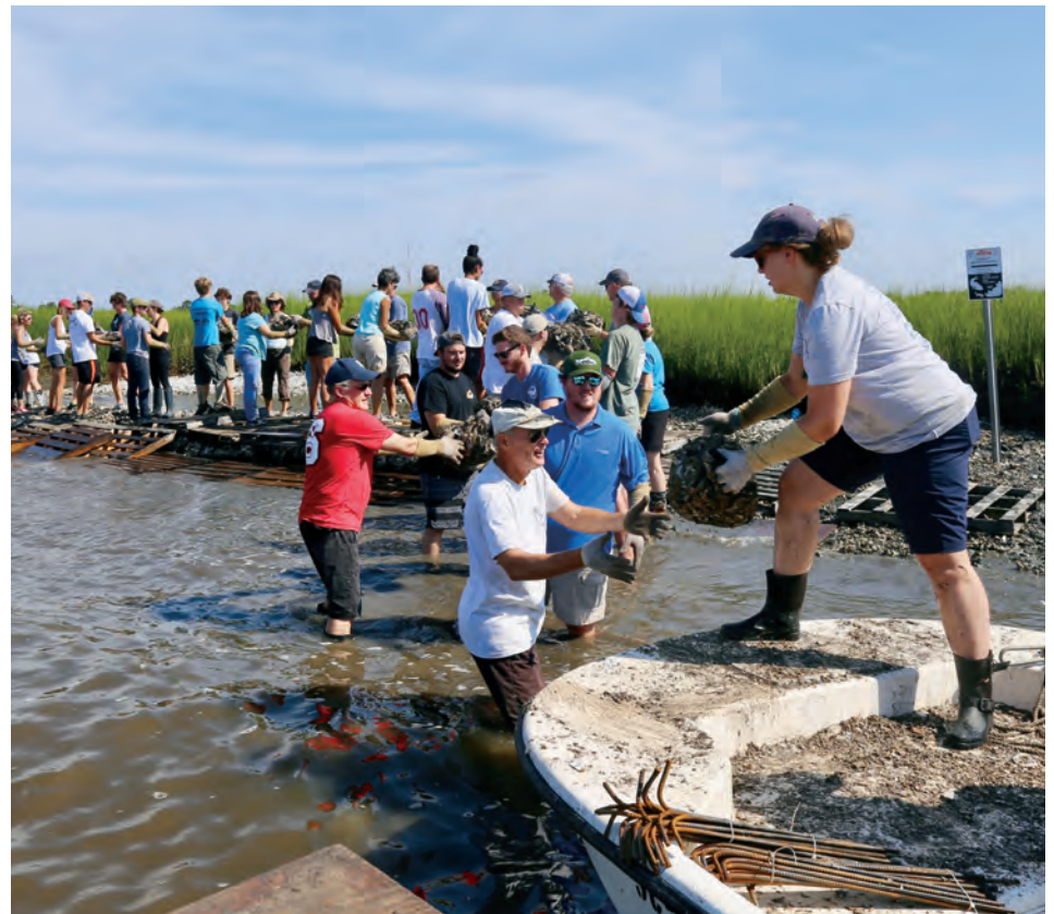
Lowcountry Land Trust has been working with South Carolina Oyster Restoration and Enhancement (a program of SC Department of Natural Resources) and the U.S. Fish and Wildlife Service to install oyster reefs—a living shoreline—at several different properties around Charleston County.
